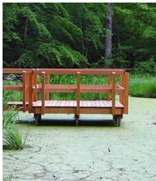
Bird-watching footbridge (Switzerland)
