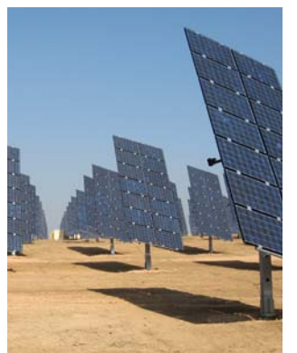
Tracked PV installation (Spain)
