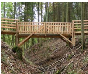
Timber bridge, Baden-Württemberg
