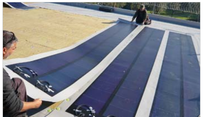
Fig. 9: Overlapping alignment of the membranes
