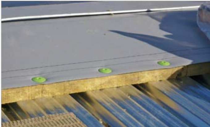
Fig. 6: Overall view of trapezoidal sheet metal, insulation and TF Membrane Professional
