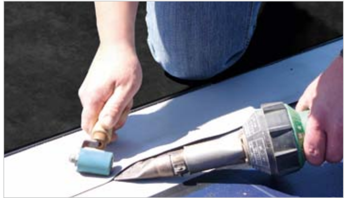
Fig. 13: Manual welding with a protection mat.
