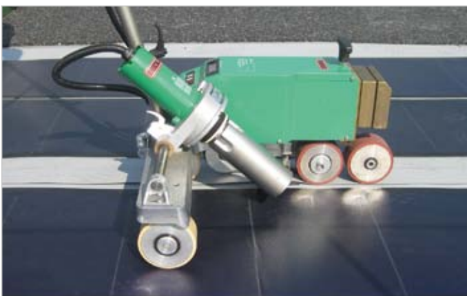
Fig. 12: Machine Welding of TF Membrane Professional
