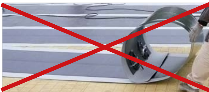
Fig. 3: TF Membrane Professional must not be rolled during installation!
