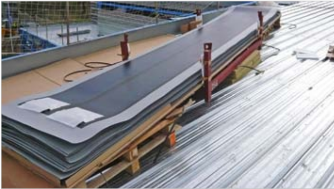
Fig. 2: On the roof, place pallet in a location that can withstand high loads.
